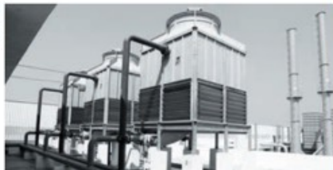
Chilling plant cooling towers New plant at Tunapundla village
